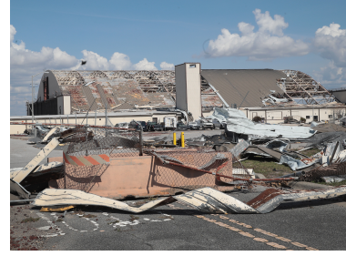
Figure 4. Destruction of Hurricane Michael on Tyn-dall
