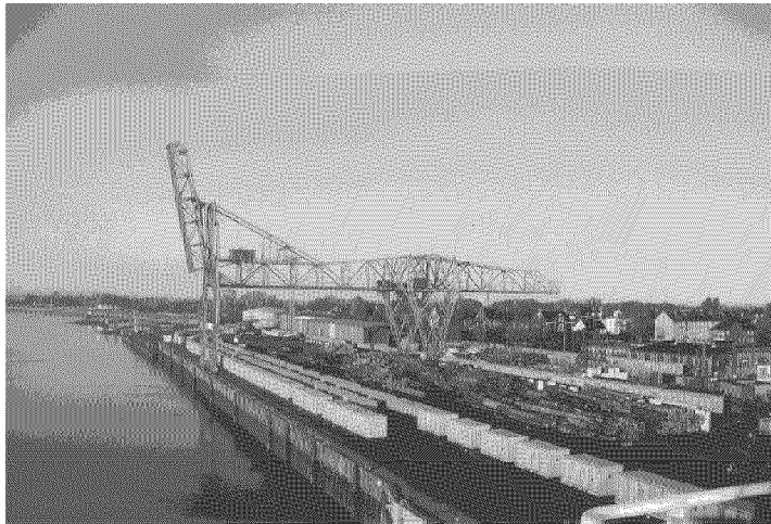
Figure 3-2. ISO Containers Being Loaded onto Railcars
