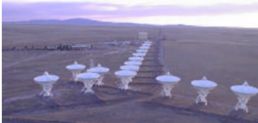
Figure 3.11 The “Y” shape of the VLA was chosen to minimize the number of (\vec{u} \vec{v}) cells not intersected by a receiver locus over a viewing period.
