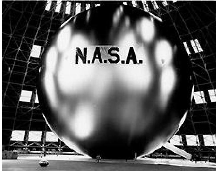
Figure 2.1 NASA Echo I Satellite
