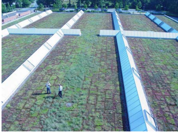
Figure 4.9 Oldenburg Bus Station. Atypical roof. Vegetated mats made with coconut fibers that later shrunk leaving gaps between the mats. Gaps filled in with mosses.
