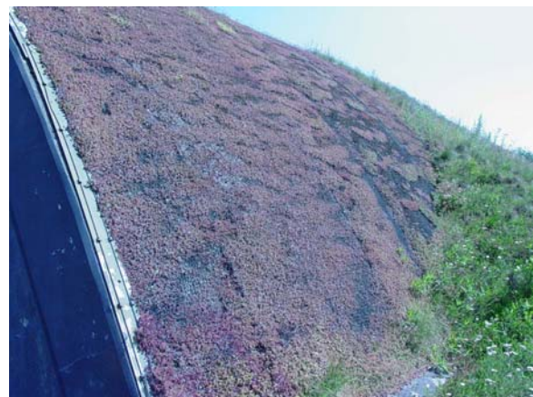
Figure 4.16 Bunker 1. The plastic sling/coil that holds the mats in place can be seen through the sparse vegetation.
