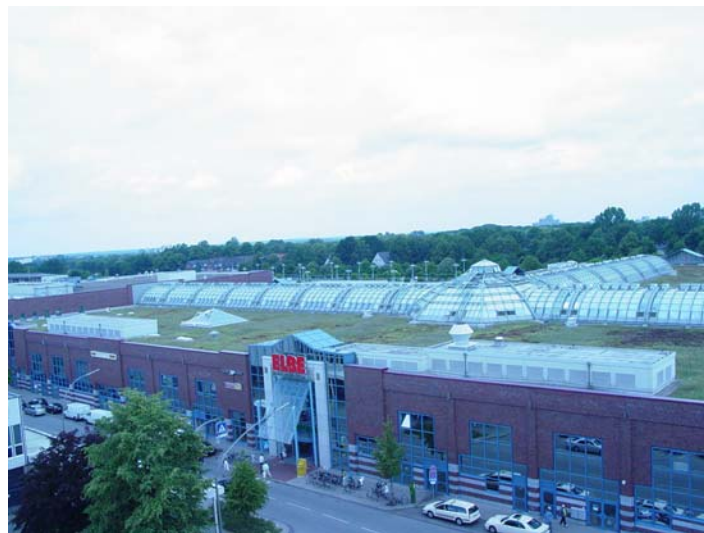
Figure 4.26 Elbe Center Department Store. The cooling benefits of the roof and the ventilation from the open skylights eliminates the need for air conditioning.
