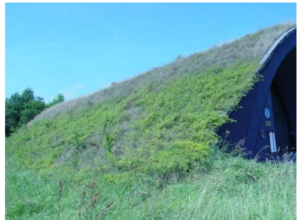
Figure 4.18 Bunker 2. Bunker 2 provides excellent camouflaging effects from overhead by sustaining grasses and other woody stemmed plants.
