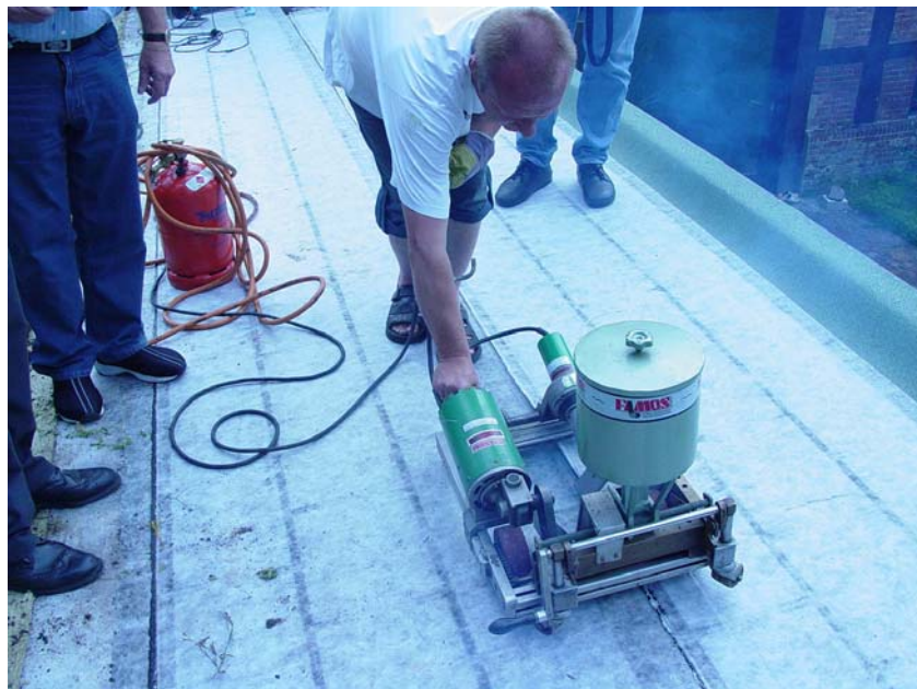
Figure 2.5 Famogreen Ret. This water proofing membrane has inherent root protection and uses gel crystals to provide water retention capabilities.
