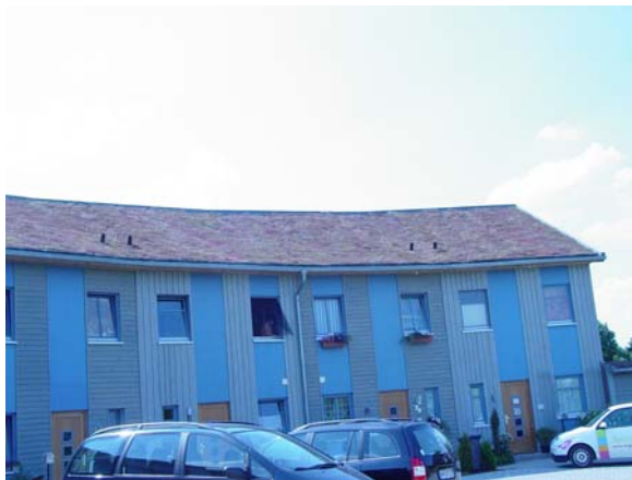
Figure 4.23 Apartment Building. The vegetation on the 2 year old apartment building was installed as vegetated mats.
