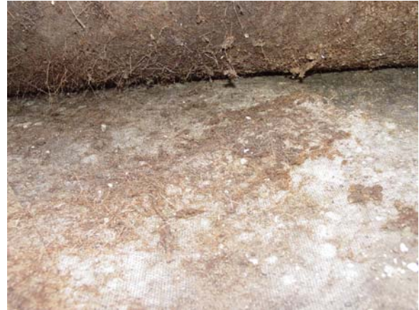
Figure 4.28 WIRO GmbH Roof. Slender sedum roots can be seen on the bottom of the vegetated mats and broken off on the Famogreen Ret membrane underneath the mats. Roots grow through the white fabric to reach the water retaining gel crystals below.
