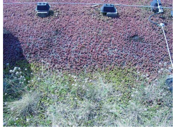
Figure 4.22 Building 3. Only sedums exist on the raised portions of the roof with no soil.
