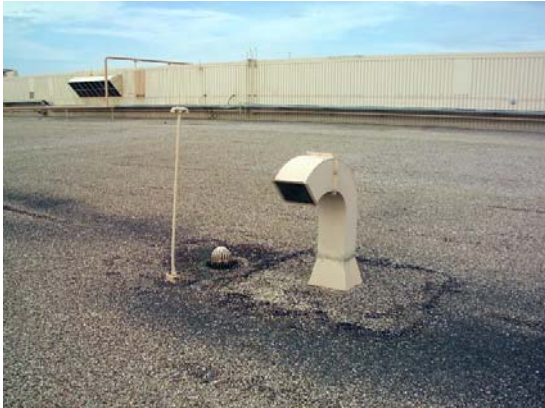
Figure 2.1 Asphalt BUR. Roof drain and vent.
