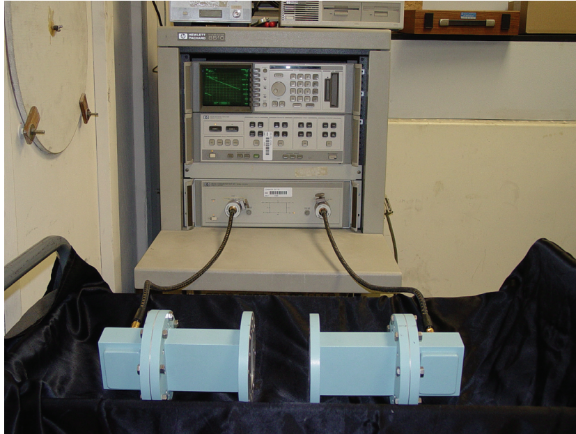
Figure 4-1. Experimental setup showing the WR284 waveguide connected to an HP8510B Network Analyzer via coaxial cables. The reduced-aperture sample holder is mounted between the waveguide feeds using precision alignment pins.
