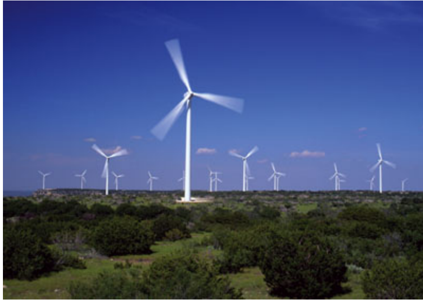
Figure 13. Trent Mesa Wind Power Facility
