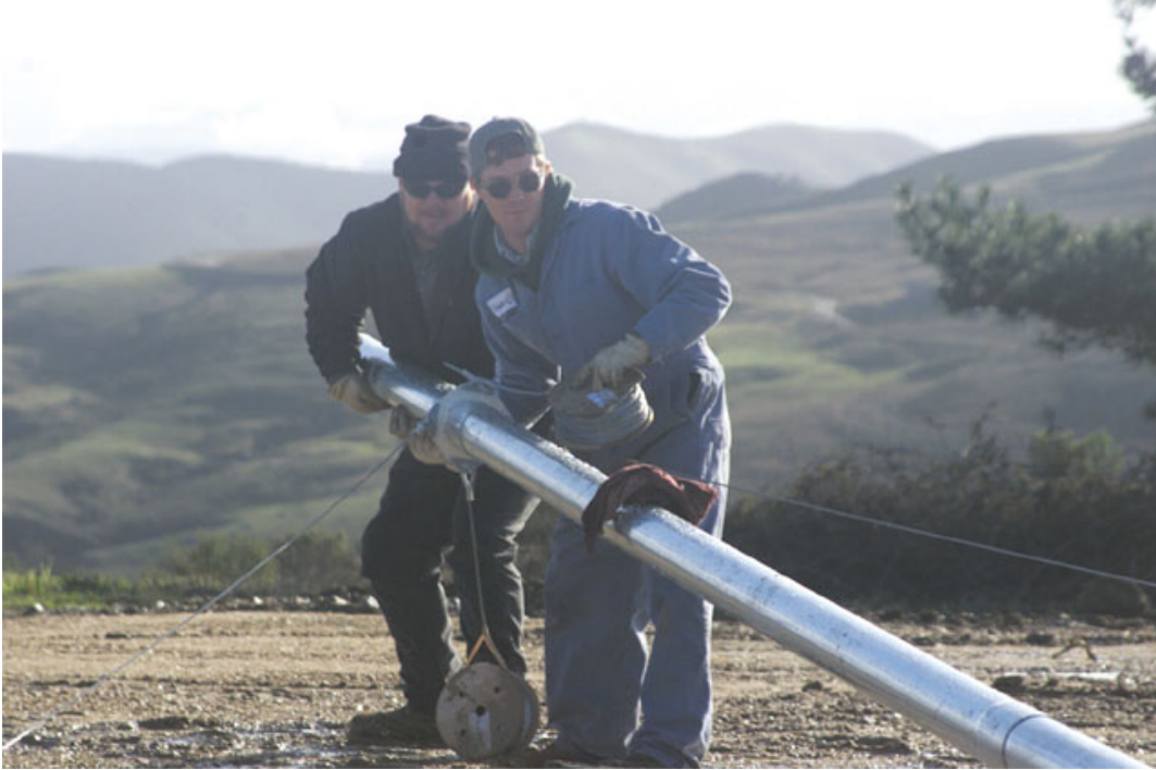
Figure 6. Anemometer Installation
