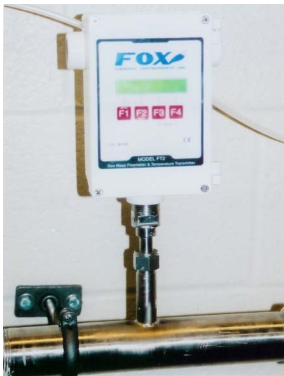
Figure 6 Fox Thermal Instruments FT2 Flow Meter
