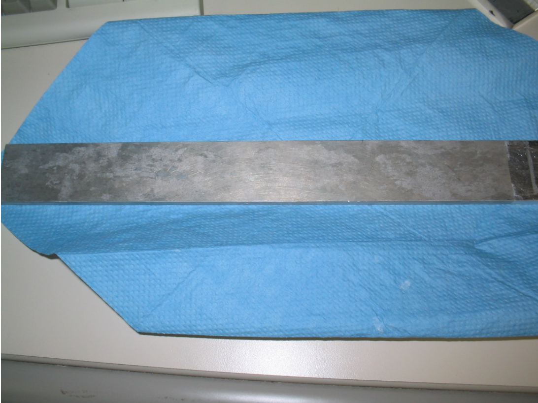
Figure 198. White/red middle notched beam after corrosion and cleaning. Lighter gray areas represent where salt deposits were present, while darker gray areas indicate a larger extent of general corrosion, due to the absence of salt deposits.
