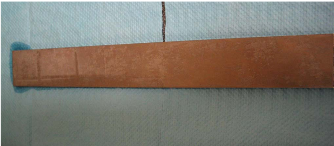
Figure 207. Front of blue/green notched beam after cleaning.
