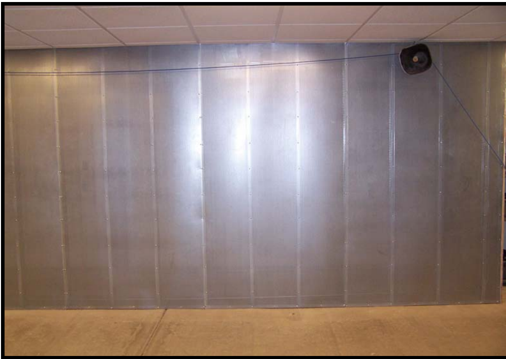
Figure 3.1 Supplied Air Wall. Air movement designed to force air contaminants down range away from instructors and shooters.
