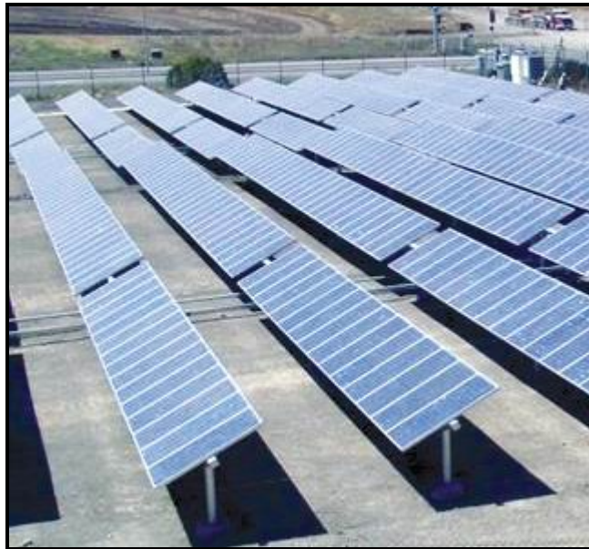
Figure 2.6. An Example of Fixed Position Solar Panels (H2-PV, 2007).
