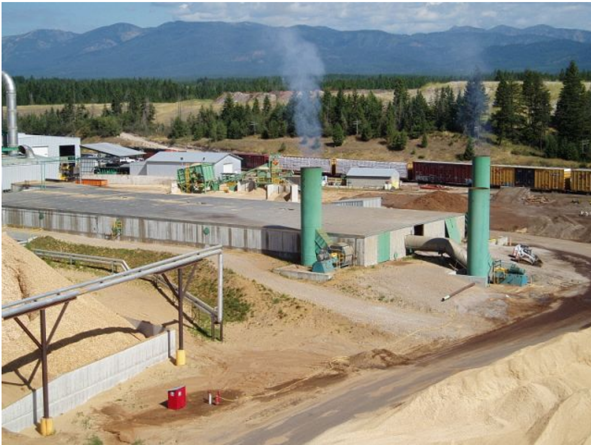
Figure 4.3. The Plum Creek Timber Company, Inc., medium density fiberboard facility biofilter in Columbia Falls, Montana (Leu, 2007).
