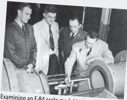
Examining an F-84 scale model in the 20-foot low speed wind tunnel in 1953.
