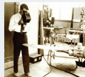
A student at the Air Corps Engineering School studies the effects of propeller vibration during the 1930's.
